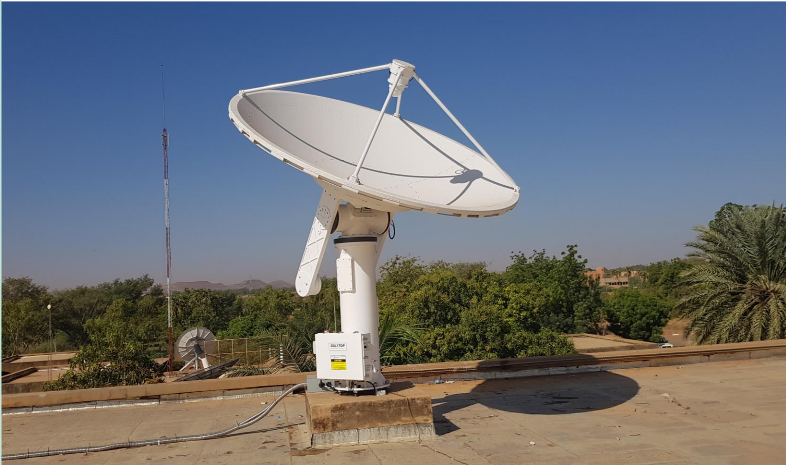
RARS station installed on the roof of AGRHYMET's building (Niamey- Niger)
