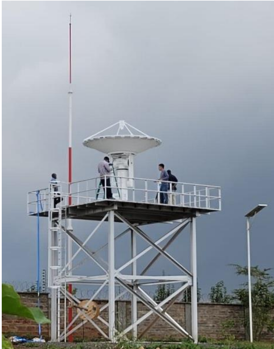
RARS station built at ICPAC's premises (Kibiko Ngong – Nairobi, Kenya)
